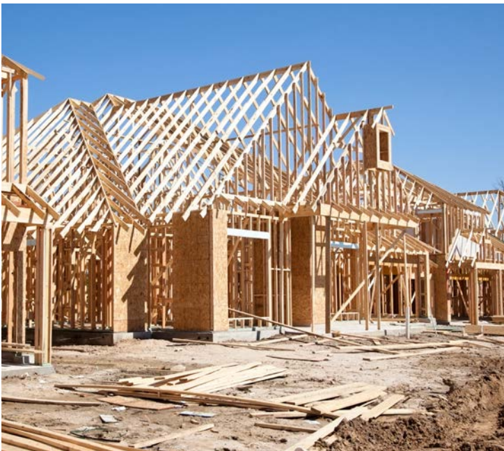
New Housing Construction (ABAG Archives)
