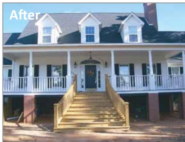
Photos (left): A house that was elevated as part of an HMGP grant funded project to mitigate repetitive loss properties in the Coral Strip Parkway. Photo courtesy of Santa Rosa County (August 30, 2010).
