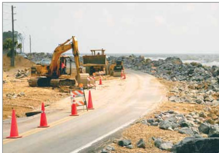
Photo (above right): Crews make emergency repairs to this damaged road after Hurricane Katrina washed away a rock sea wall that was built to protect it. After the storm, many homes and roads were flooded or damaged and residents were displaced. FEMA Photo/Marvin Nauman (August 31, 2005, Cape San Blas, Gulf County, Florida).
