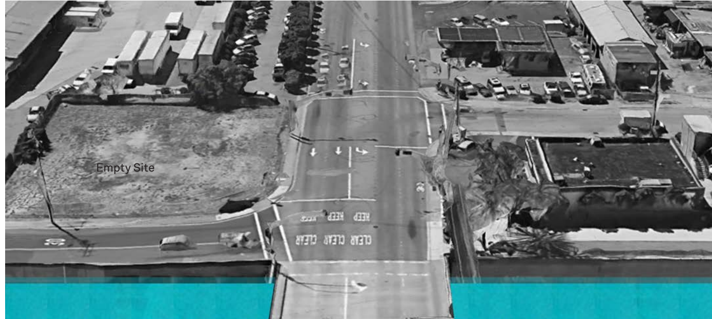
Existing storm water pipe below Spurce St
