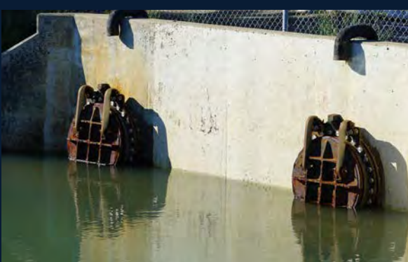
Existing pumps, tide gates, and outfalls
