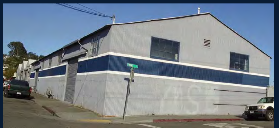
Industry and commercial businesses throughout low-lying area
