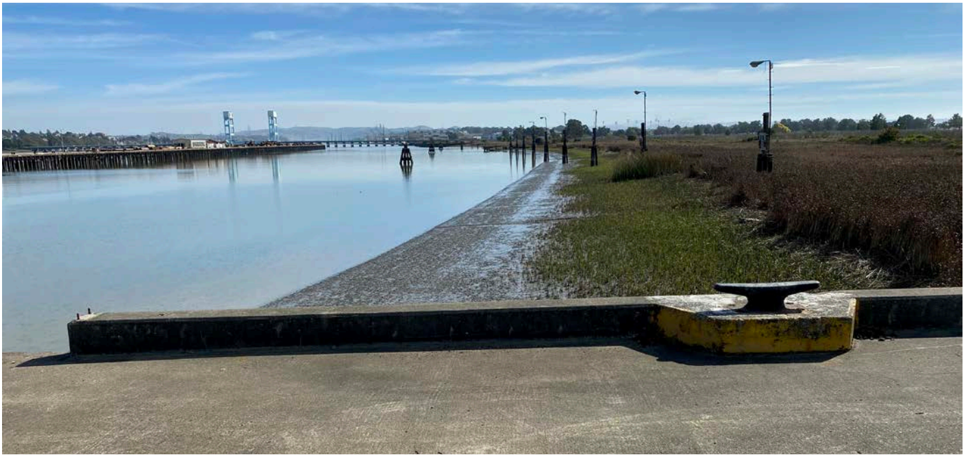
Mare Island Straight looking toward the Vallejo Causeway Bridge.
