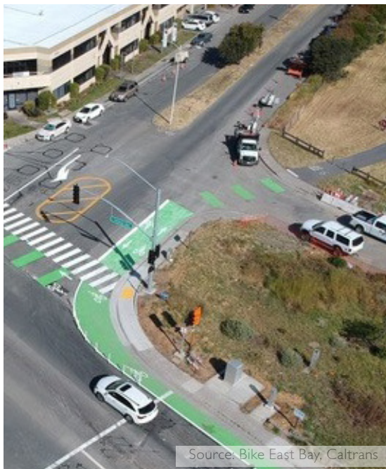
Green paint, bicycle conflict striping, flex posts, and high visibility crosswalks improve the bicycling, walking, and wayfinding approaching the Bay Trail in Richmond, CA. The paint and posts are near-term solutions that can be upgraded to more substantial, separated facilities.
