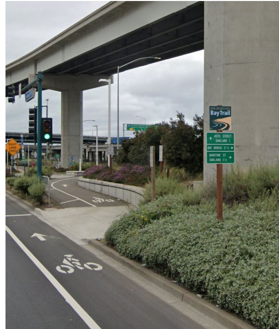
Bicycle lanes on Shellmound Ave in Emeryville, CA connect cyclists from downtown to the Bay Trail. Separated bicycle lanes with physical barriers are preferred to make this experience more comfortable for all users.
