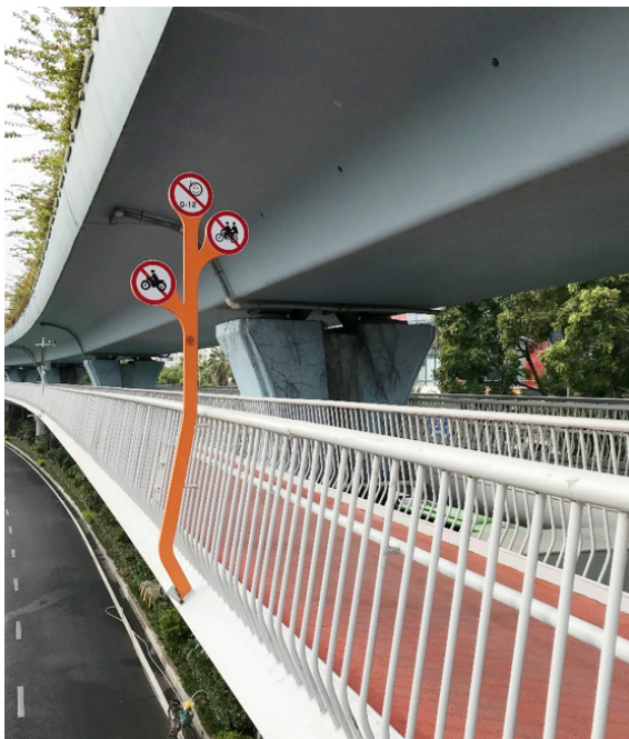
Structures should relate to each other and feel comfortable for all users.
