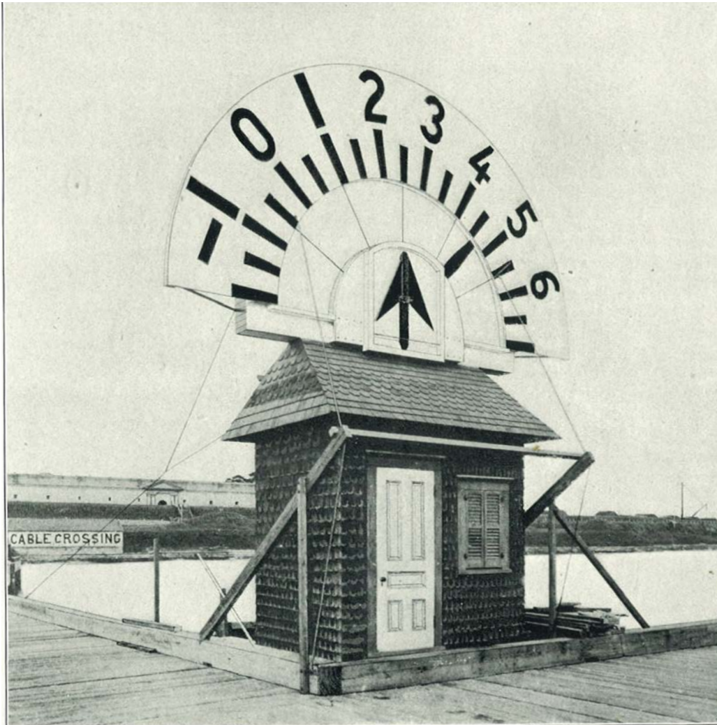
Tidal Indicator, New York Harbor, ca 1900. US Coast Survey/NOAA. A series of tidal indicators were used along US coastal cities to alert incoming vessels of predicted tidal levels. A replica was erected on Alcatraz facing the Golden Gate.
