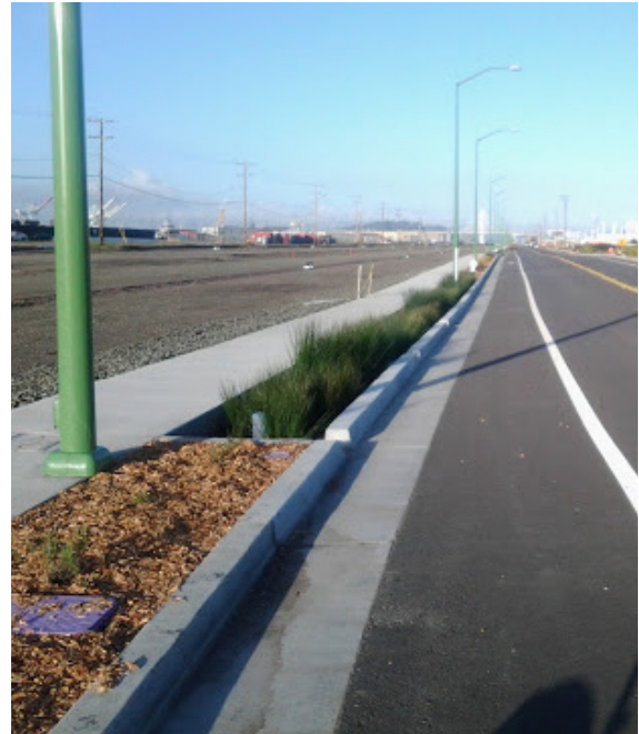
Flow through planters and other types of green infrastructure help control storm runoff and reduce the need for supplemental irrigation.
