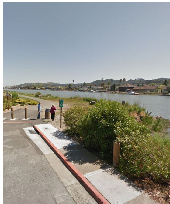
A bicycle route on a residential, dead-end street connects the adjacent residents to the Bay Trail along the Corte Madera Creek in Larkspur, CA. On-street facilities should only be considered on low volume streets and separated facilities are preferred.
