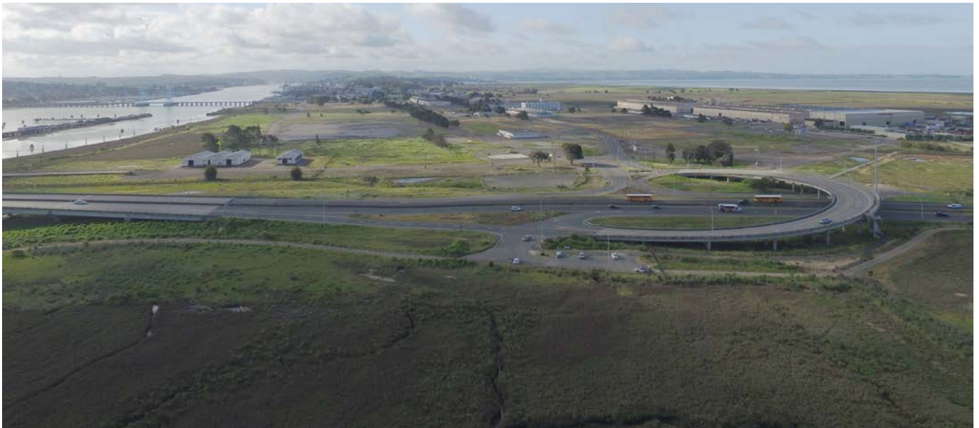
Northern end of Mare Island at S37 interchanges - showing parking and overlook
