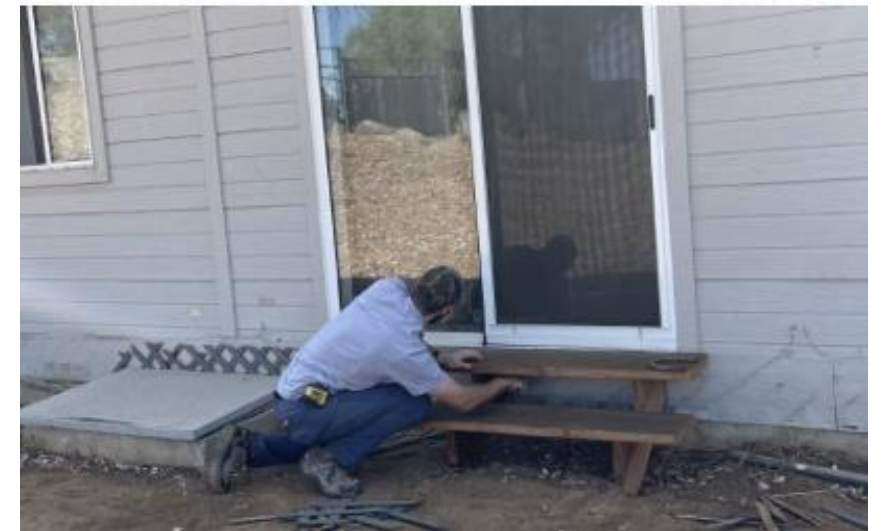
Removing the Combustible Skirting
