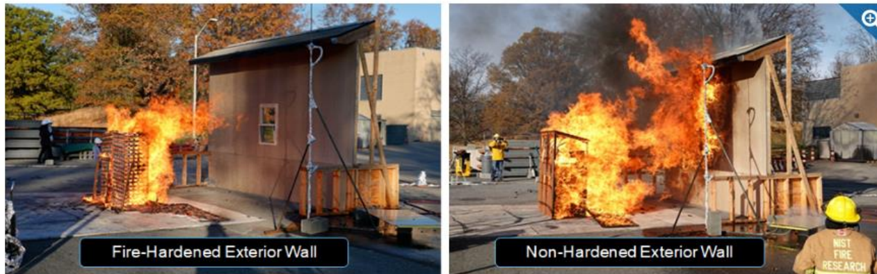
Photos from NIST experiments show the effects of a burning shed located 15 ft from the primary structure.
