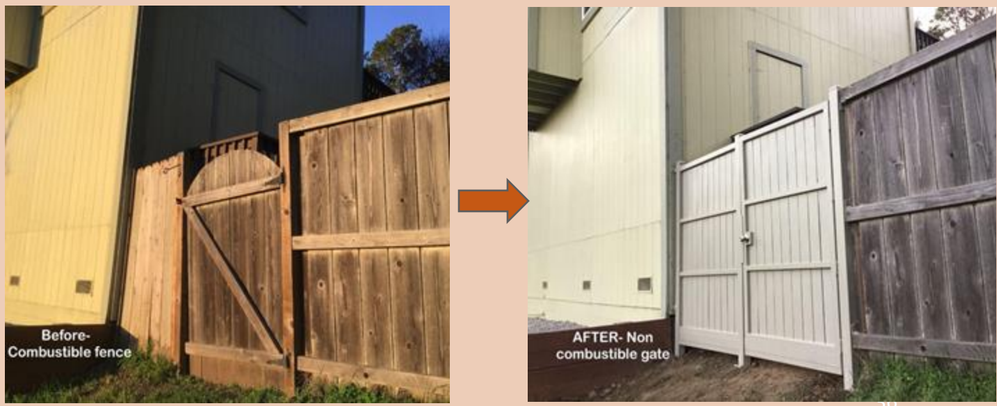
Combustible to Non-combustible Fence Connections
