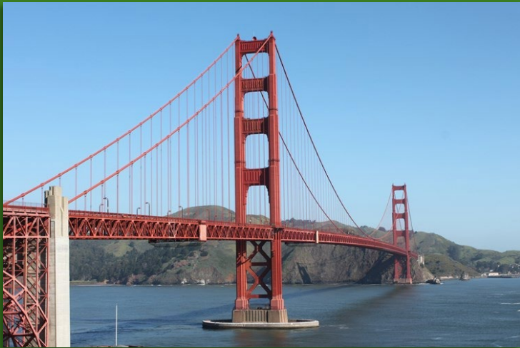
Golden Gate Bridge
