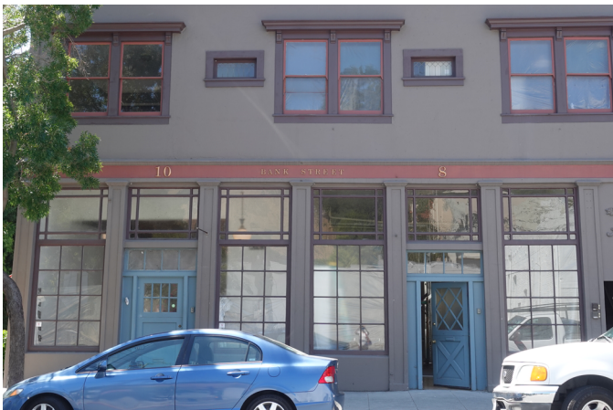
Example of a Maker Shopfront.
