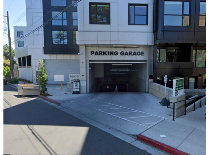
Minimized loading and garage access on a residential street
