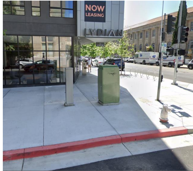
Most unfortunate placement of utility boxes: Lydian, Oakland
