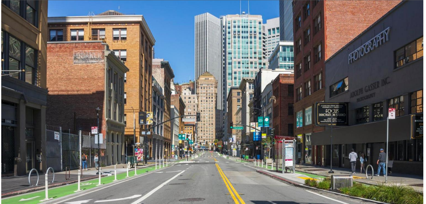
SPUR: Office to Housing Conversion (2022) (Photo: Sergio Ruiz)
