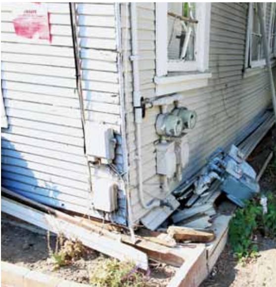
Cripple wall and gas connection failure. South Napa Earthquake. Photo credit: EERI - Petros Keshishian
