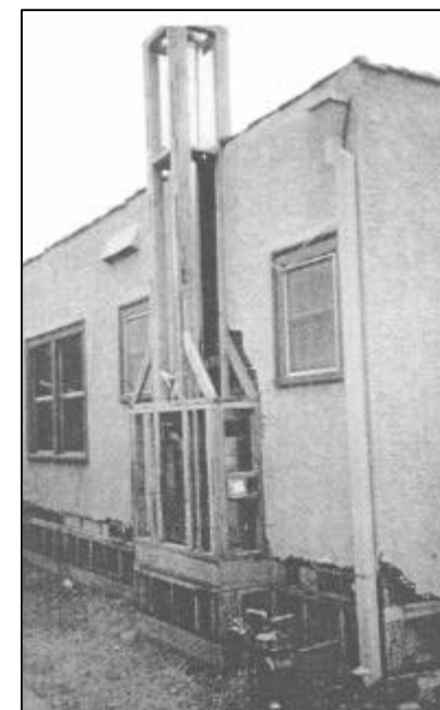
Fig. 7.3 Chimney Replacement
