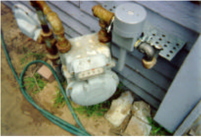
Fig. 7. 7 Automatic Shutoff Valve
