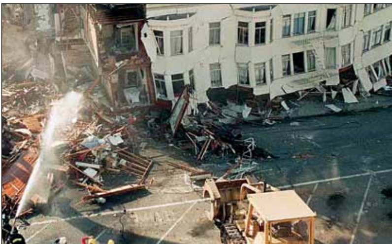
Soft Story Failure, Loma Prieta Earthquake
