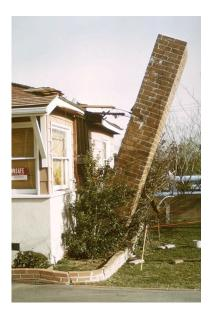
**Nonstructural components.** Any part of a building that's heavy, brittle, or loosely attached, even if it carries no structural loads, is vulnerable to earthquake damage. The heavy parts – chimneys, brick veneer, concrete cladding panels – can be life threatening. The gas lines and gas-fired equipment can start fires. The rest – light fixtures, plumbing and sprinkler lines, HVAC equipment, shelving, and so on – can take a building out of service, disrupting operations and delaying recovery.
