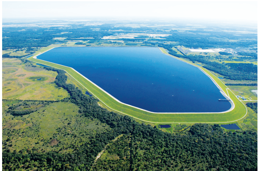
Figure 4.1. During the rainy season, excess water from the Tampa Bypass Canal and the Alafia and Hillsborough Rivers is sent to the C.W. Bill Young Regional Reservoir. This water helps bridge the gap during the dry season.
