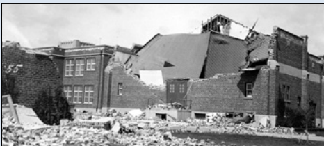
One of the schools damaged in the 1933 Long Beach earthquake
