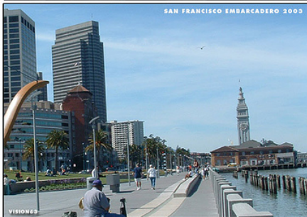
Demolition of San Francisco Embarcadero Freeway led to a walkable pedestrian boulevard
