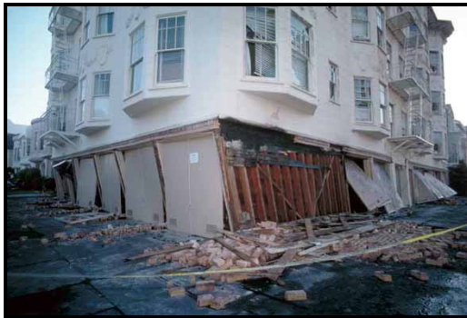
Damage to Housing in 1989 Loma Prieta Earthquake
