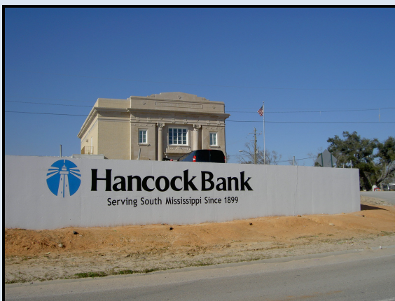
Hancock Bank repair in Mississippi following Hurricane Katrina was based in part on regional commitment and customers in southern Mississippi.
