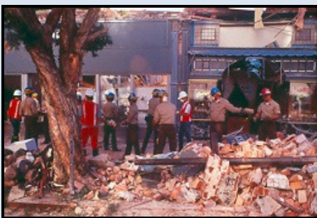
Pacific Garden Mall in downtown Santa Cruz following 1989 Loma Prieta earthquake
