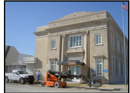
Hancock Bank repair following Hurricane Katrina, Pass Christian, Mississippi
