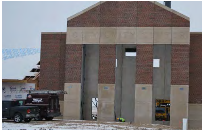
Palo City Hall/Community Center under construction
