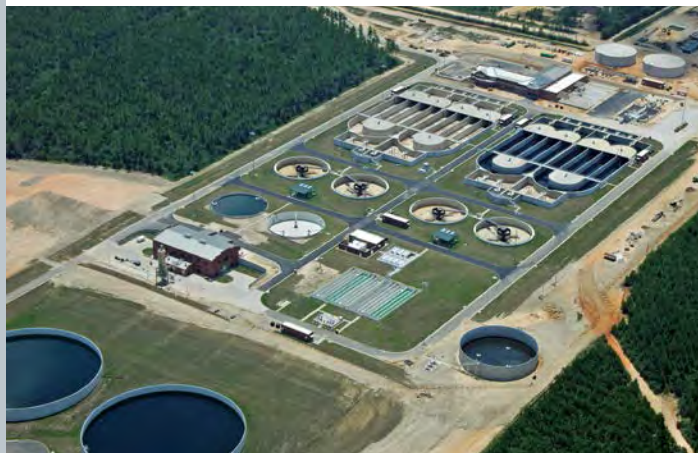
Central Water Reclamation Facility, Escambia County, FL
