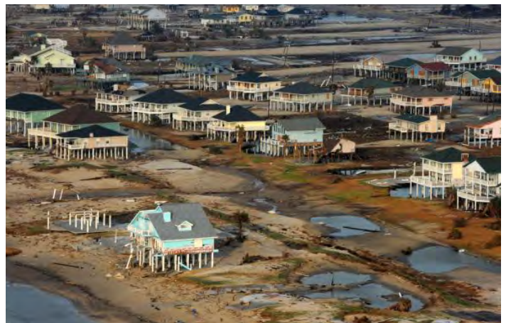
Damaged homes in Bolivar Peninsula after Hurricane Ike
