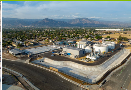
EAST VALLEY WATER DISTRICT HIGHLAND, CA SUPPLY
