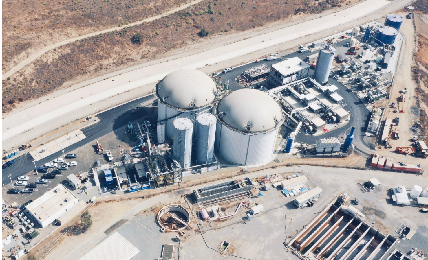
Rialto Bioenergy Facility
