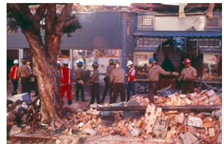
Pacific Garden Mall in downtown Santa Cruz following 1989 Loma Prieta earthquake
