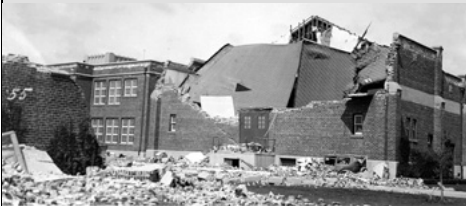
School damaged in the 1933 Long Beach earthquake
