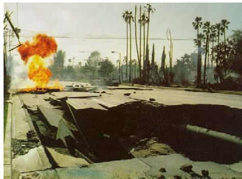
Damage to road in Northridge earthquake
