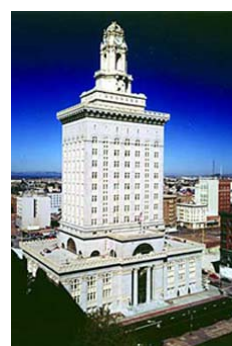
Oakland City Hall retrofitted after Loma Prieta earthquake
