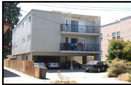
Soft Story Apartment in Oakland
